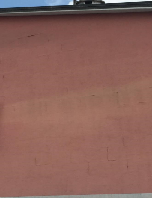
Low-quality and/or poorly applied adhesive
